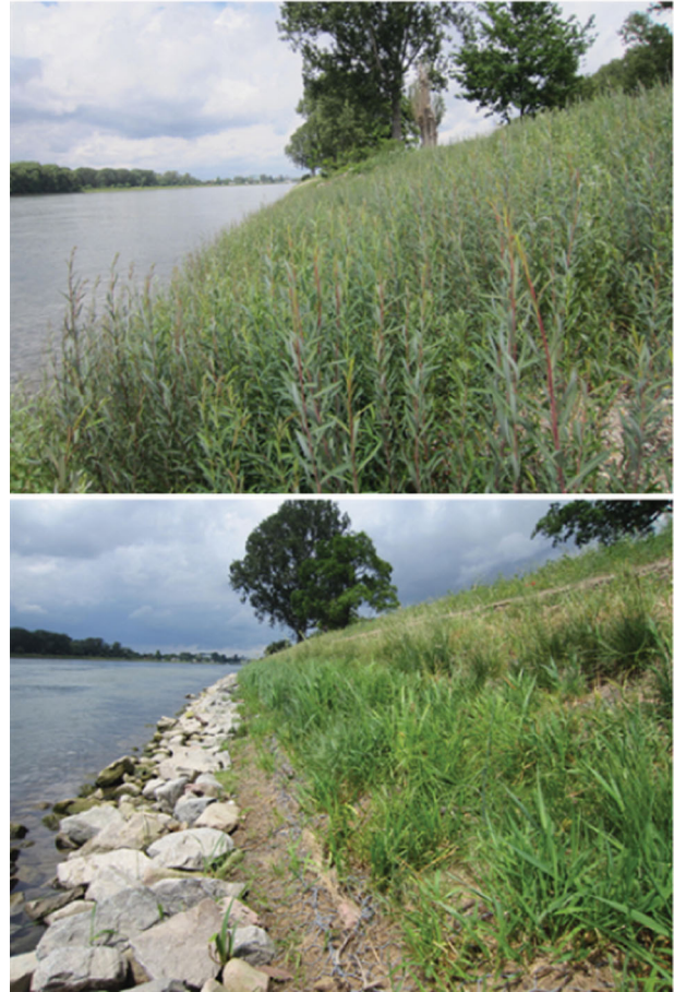
Figure 1. Two examples of technical-biological bank protections on the Rhine (upper picture: willow brush mattresses, lower picture: vegetated gabions, both 7 months after installation).
